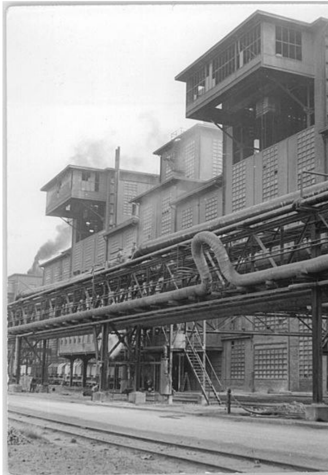
Carbide building, Schkopau
